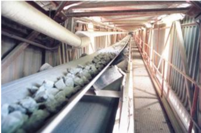
Figure: 1. Raw limestone (calcium carbonate) from the Northern Cape
