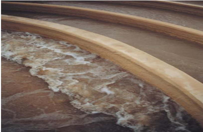
Figure: 2. Flocculators or baffled channel conditioning bays used in Rand Water.
