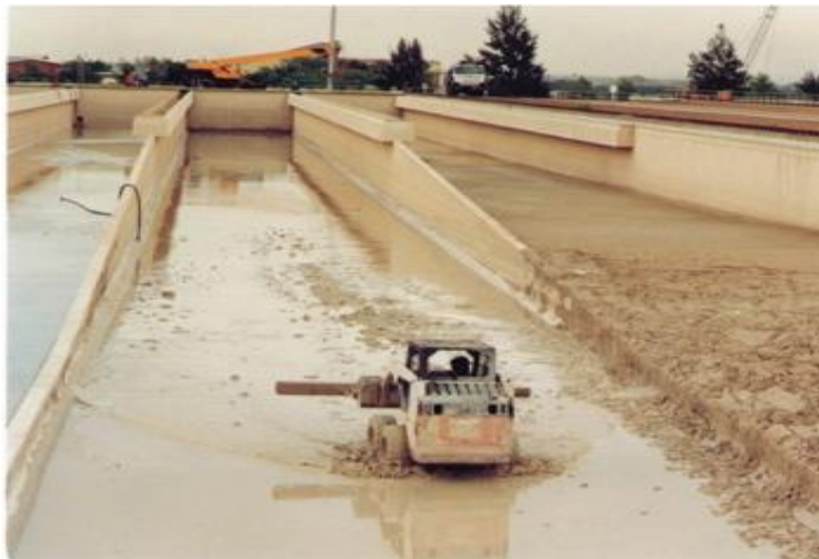
Figure: 4. Removal of dry sludge
