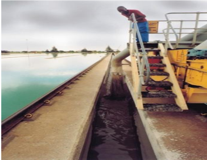
Figure: 3 Sedimentation tank
