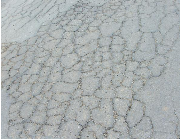
A1: Crocodile Cracks
