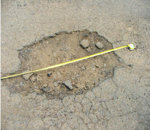
A5: Surface Failure
