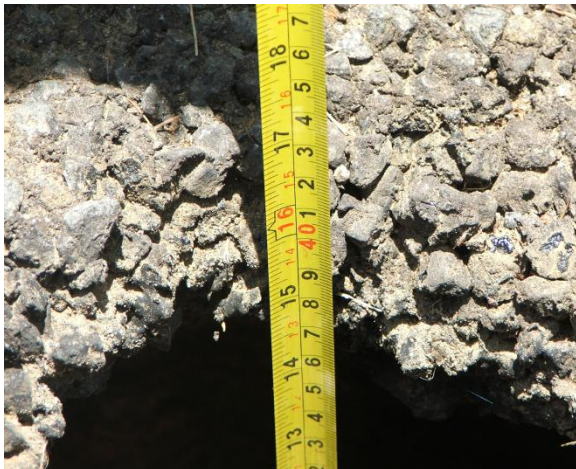
A3: 150mm Deep Pothole
