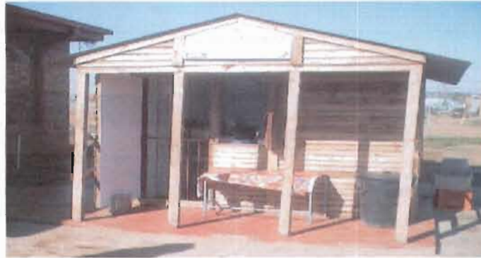
Figure 5.1: The kiosk erected for the school feeding intervention from outside
