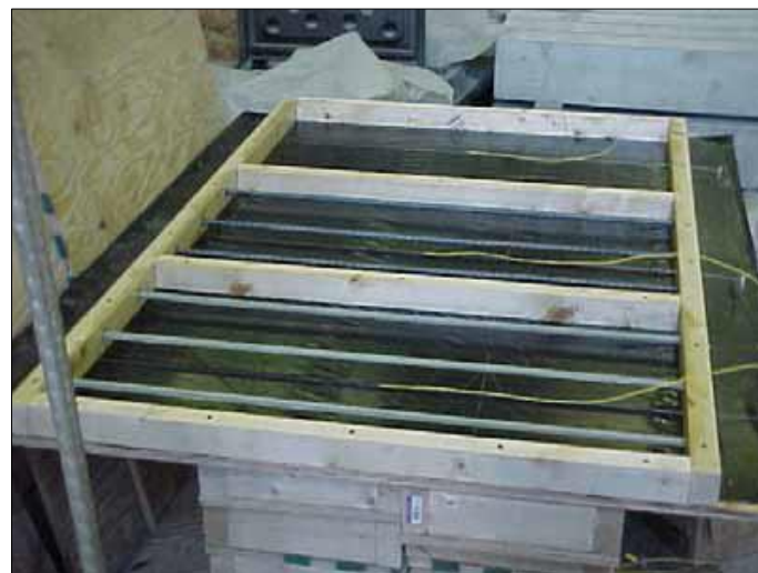
Figure 2-21 – Concrete slab moulds (Henderson, 2005)
