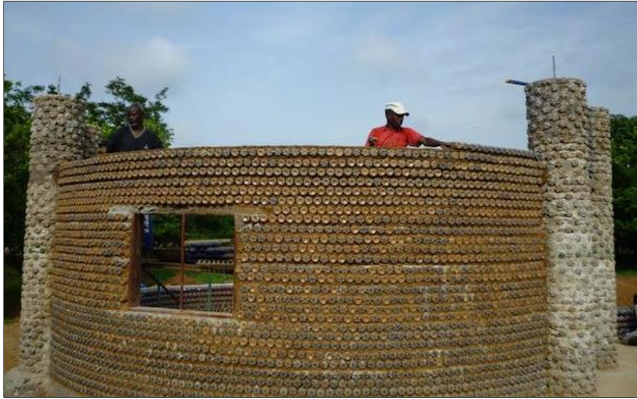
Figure 2-12 – PET bottles used in construction with cement paste (Turner, 2015)
