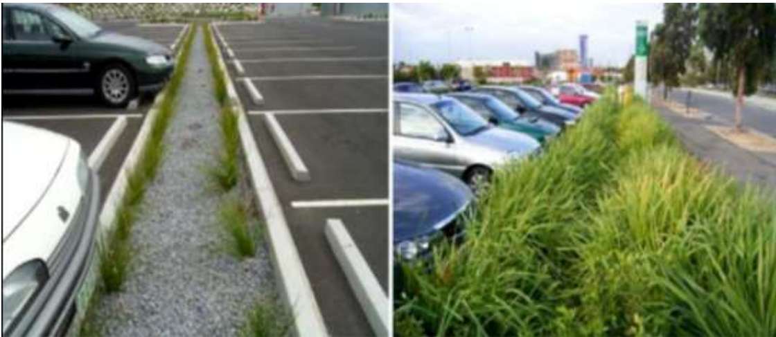
Figure 2.7: Infiltration trenches surrounding car parks (WSUD, 2005)
