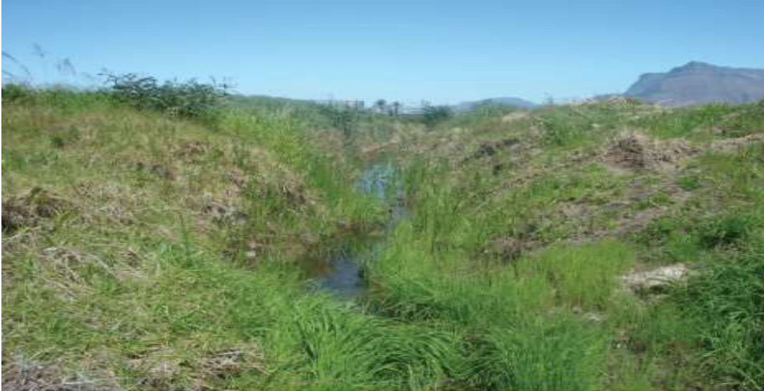
Figure 2.5: Vegetated filter (WRC, 2013).
