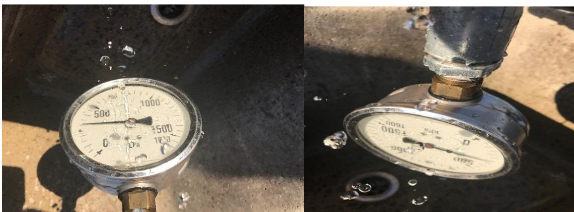
Exhibit 5: Pressure in Ext 10 measured (3 bars)
